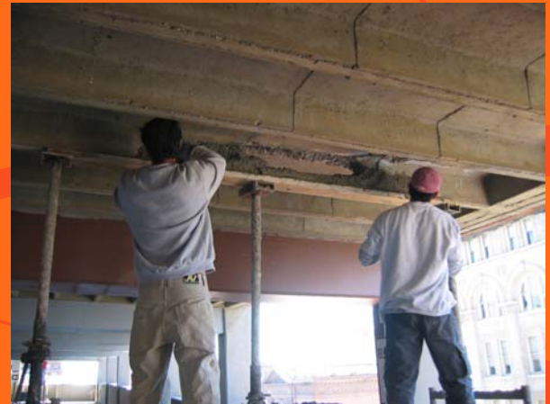
Picture: Form work in place while applying overhead repair mortar.
