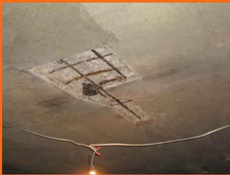
Picture: Overhead repair area prepared prior to material application
