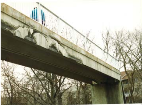
Spalled concrete on vertical and overhead surfaces
