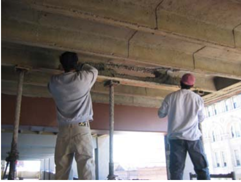
Form work in place while applying repair mortar
