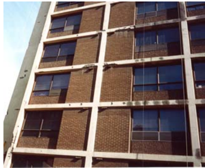
Spalled concrete on vertical and overhead surfaces
