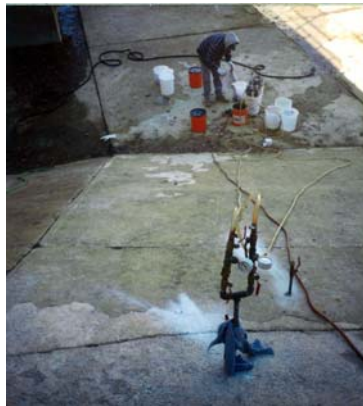
Water Intrusion Being Repaired
