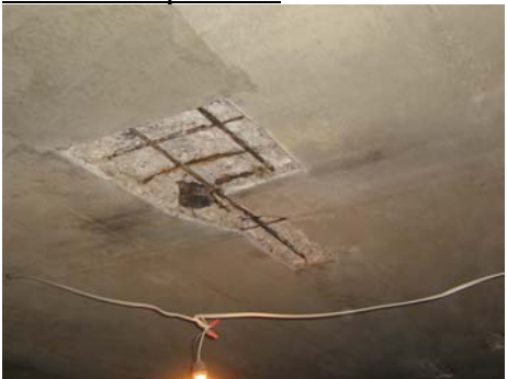
Properly prepped overhead area prior to application of repair products
