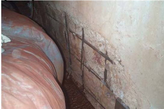
Examples of Concrete Spalls in need of repair
