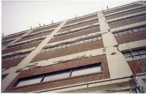
Examples of Deterioration of Concrete
