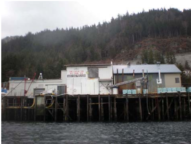
Figure 9: Ketchikan, AK – a Trident Seafood processing facility sites on a timber pile structure. Severe deterioration of the piling was threatening the facility. Restoration was completed with the fiberglass jacket system without needing a plant shutdown.
