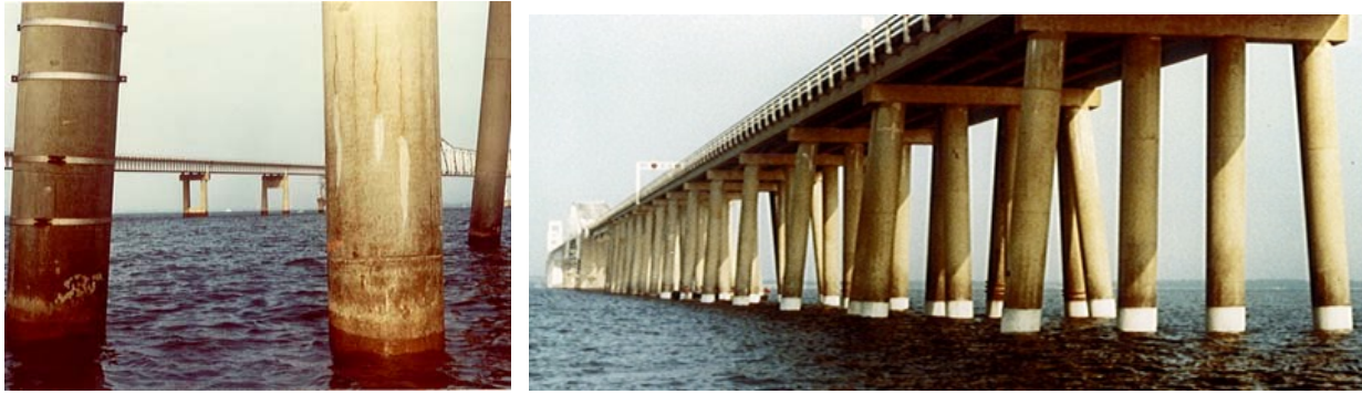
Figure 6: Piles under the Chesapeake Bay Bridge showed extensive scouring due to conditions (Left). On the right, you can see the Bridge after the restoration has been completed.
