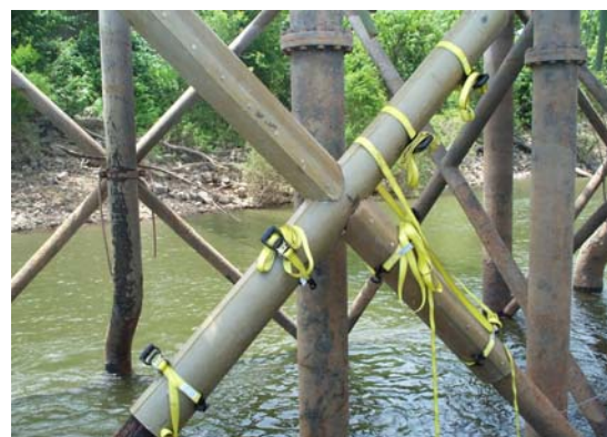
Figure 10: Inland Steel Water Intake System before and after being restored with fiberglass jackets.
