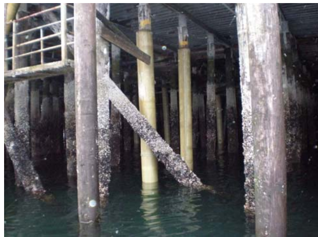
Figure 9: Ketchikan, AK – a Trident Seafood processing facility sites on a timber pile structure. Severe deterioration of the piling was threatening the facility. Restoration was completed with the fiberglass jacket system without needing a plant shutdown.
