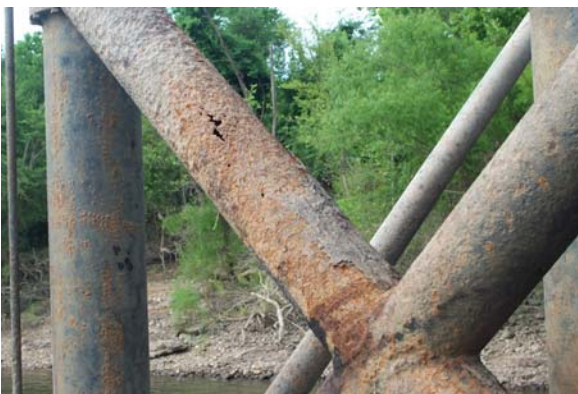
Figure 10: Inland Steel Water Intake System before and after being restored with fiberglass jackets.
