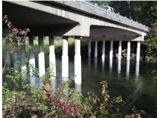
Figure 1: A completed Fiberglass Jacket Restoration
