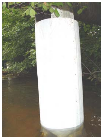
Figure 12: Steel H Pile repaired using a round fiberglass jacket.
