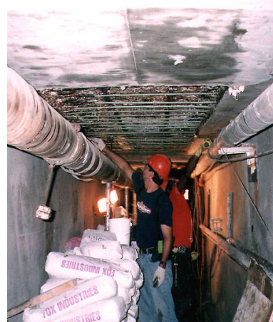
Priming Reinforcing Steel
