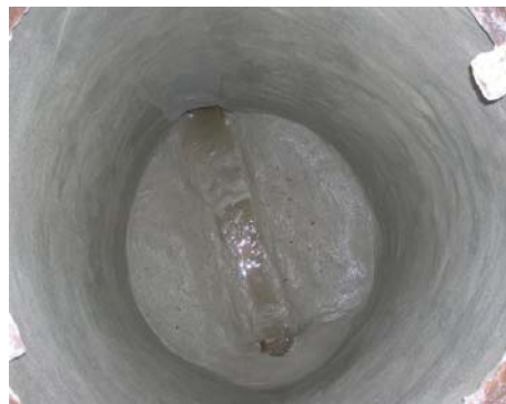
Ready for Top Coat
