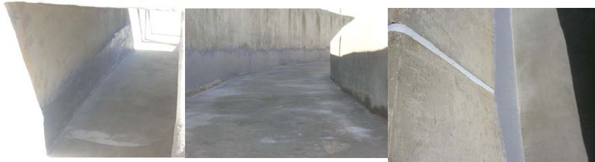
FX-472 Is Used to Fill in Bug Holes
