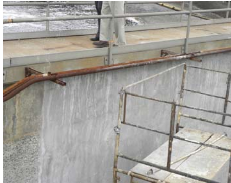
Larger View of Repair Area
