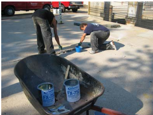
Application of FX-752 Bonding Agent
