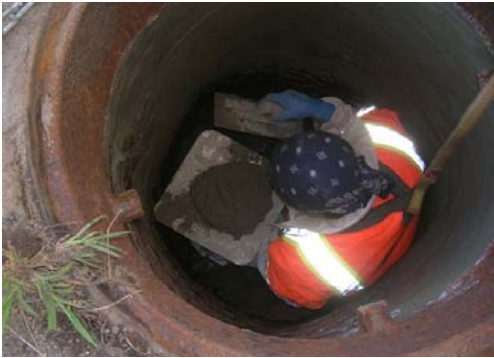
Before and After Application of FX-262
