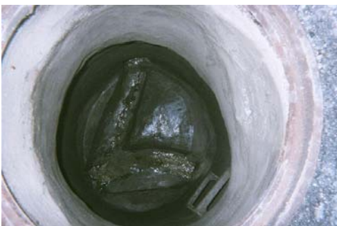
After Application of FX-293, no Top Coat Required.
