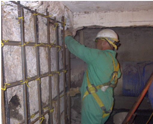
Cleaning Reinforcing Steel
