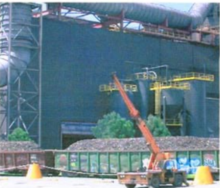
FX-509 Walnut Brown was used to coat existing building. Color was blended by Fox Industries to match new steel panels on recently installed addition.
