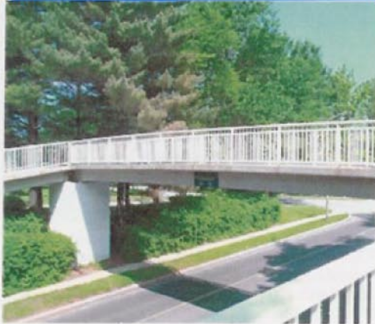
Cedar Lane Pedestrian Bridge needed new railings, deck rehabilitation, bearing work, structural repairs and appearance upgrades.
