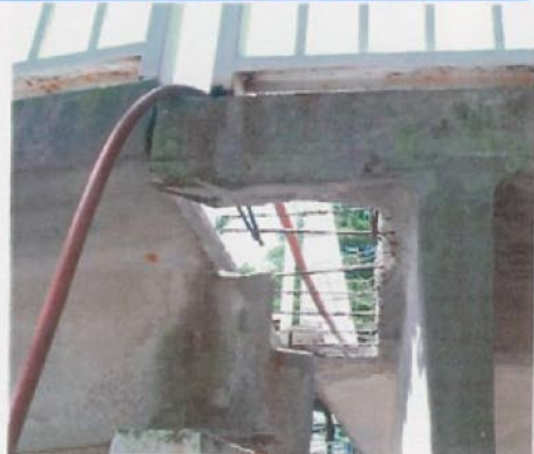
Underside view of joint area after removal of deteriorated concrete. Area was formed and poured with FX-32 Concrete Mix.
