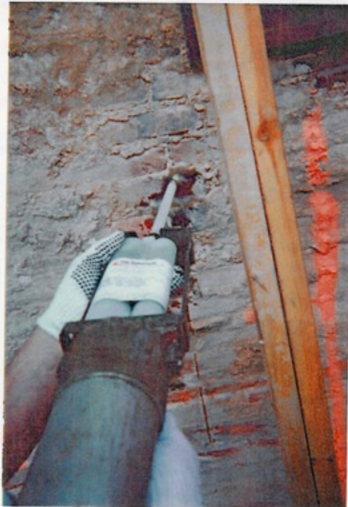
Larger voids are filled with FX-715 Hydro Ester® Non-Sagging Consistency.
