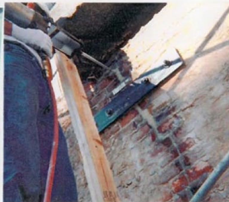
Using the static mixing heads eliminates the need to premix the injection epoxy.
