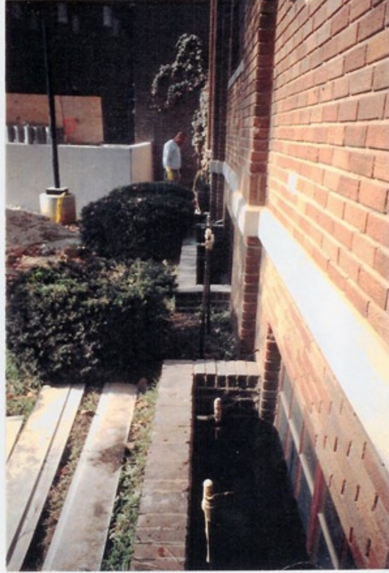
After all pipes have been pumped and removed, the pipe holes are patched with FX-922 Plug & Fast Set.
