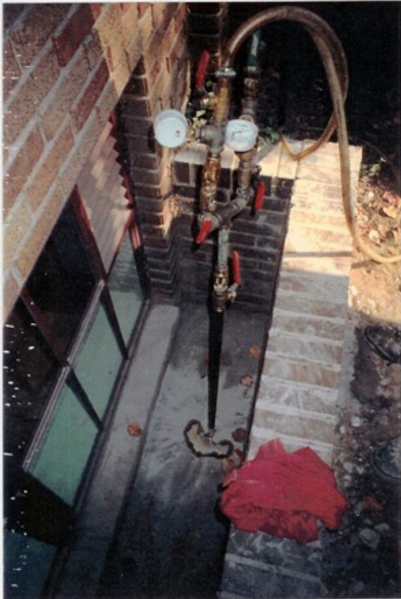
Gauges on the pump hoses allow the technicians to monitor the FX-III Jet Set during the pumping process.
