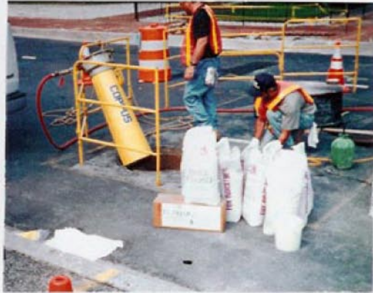
FX-408 Epoxy Zinc Rich Primer, FX-792 LP Bonding Agent, FX-228 Non-Shrink Grout, and FX-253 Reinforced Polymer Mortar are used to resurface ceiling and walls of vaults.
