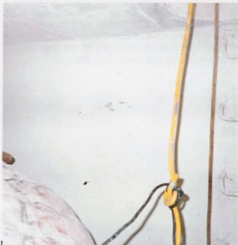
Close up view of completed wall section.
