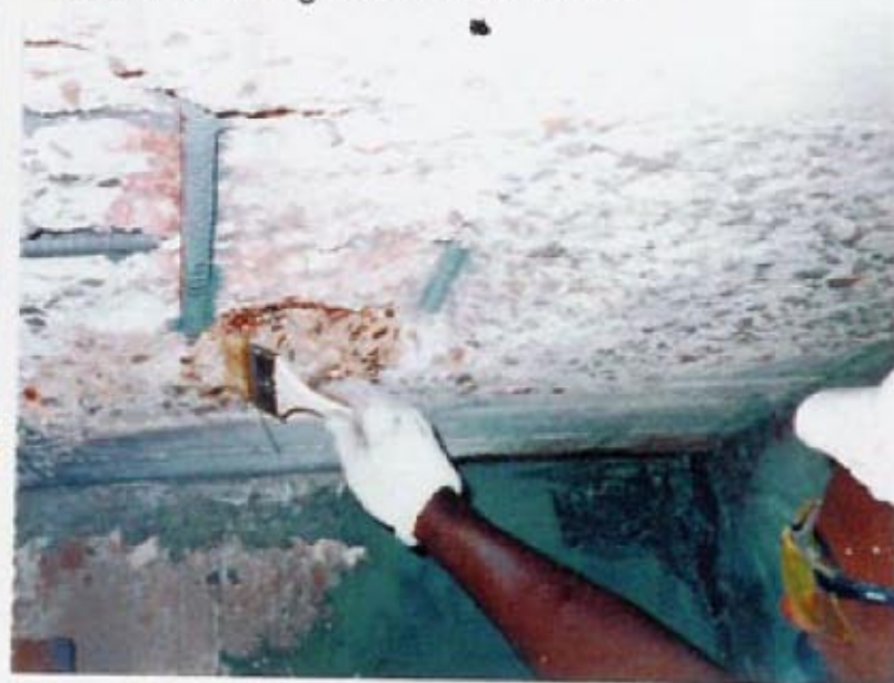
FX-408 Epoxy Zinc Rich Primer, FX-792 LP Bonding Agent, FX-228 Non-Shrink Grout, and FX-253 Reinforced Polymer Mortar are used to resurface ceiling and walls of vaults.
