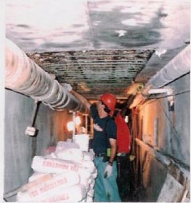
FX-408 Epoxy Zinc Rich Primer is applied to Existing reinforcing steel.
