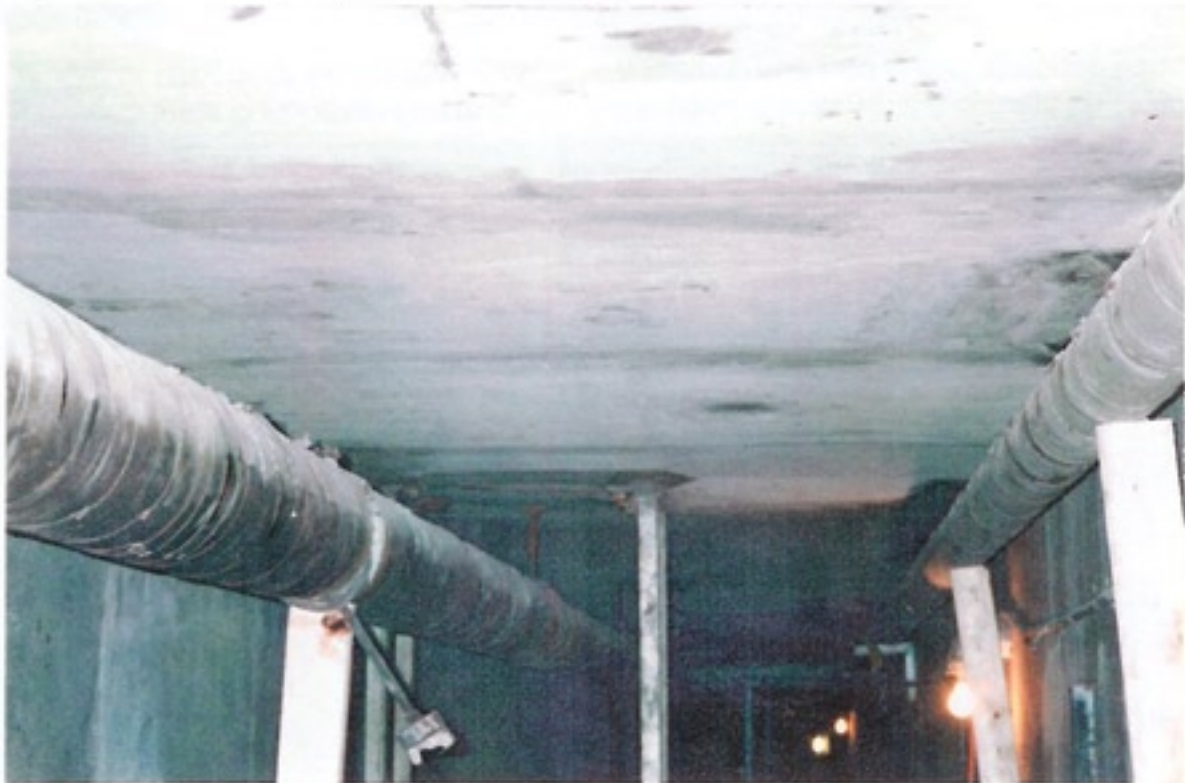
View of completed ceiling section
