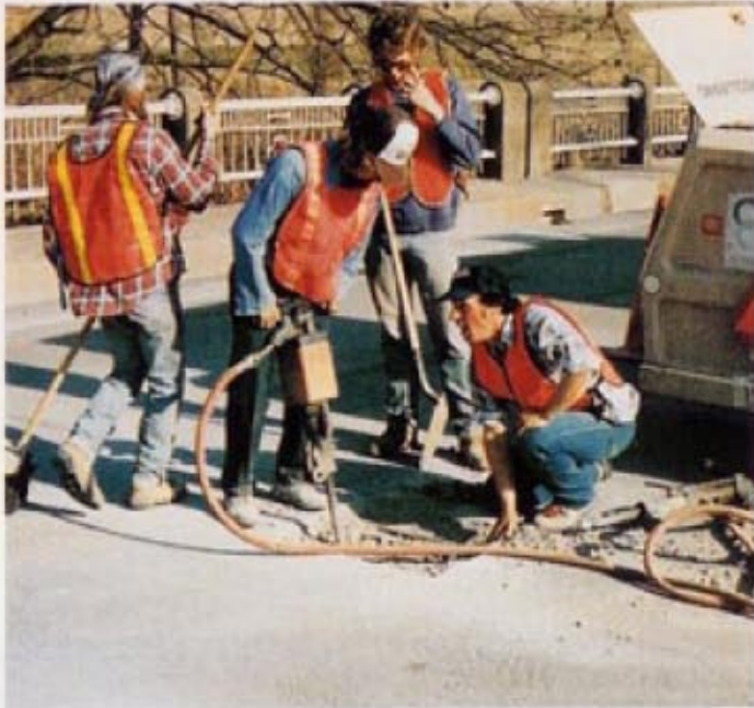
Potholes are squared off and deteriorated concrete is removed.
