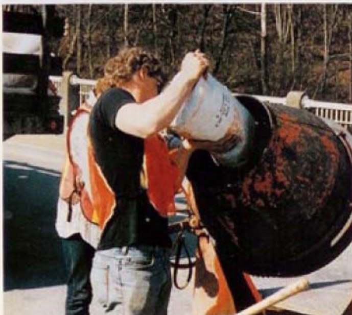
FX-928 is mixed in small portable mixer. Just add water and mix to desired slump.
