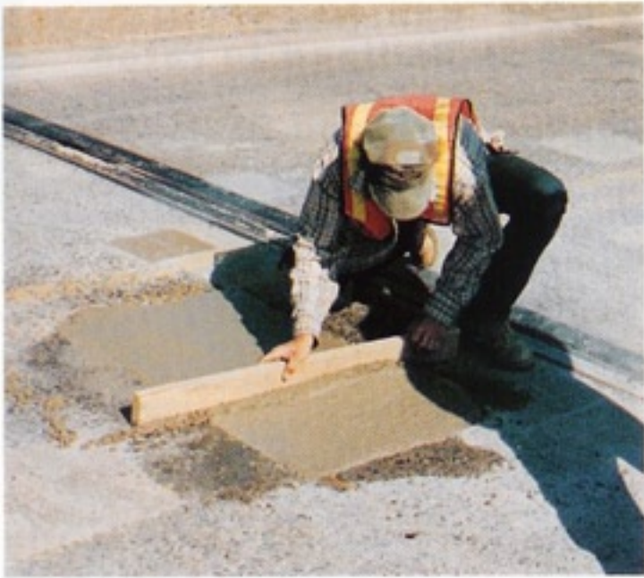
FX-928 is easily screeded by hand into place ready to finish.
